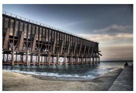
The mineral loading dock, popularly known as "Cable Inglés", is situated at the pier, in the terminal of a branch of the railway. It is an example and a masterpiece of architecture of the iron in the early twentieth century. Its construction concluded in 1904. Eclectic style characterized by the use of new materials, followed the guidelines of the school of Gustave Eiffel. In 1998 it was declared Cultural
